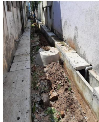
Figure 7-8 Utilities Connected to UGD
