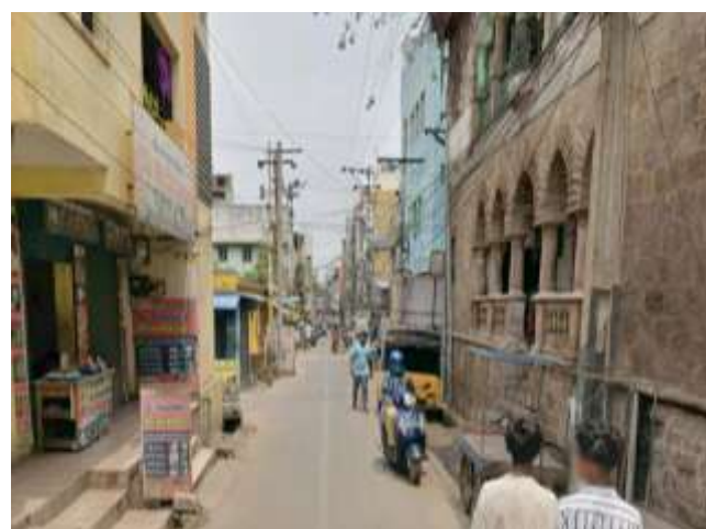
Figure 2-10 Town hall road - Commercial development near old heritage buildings
